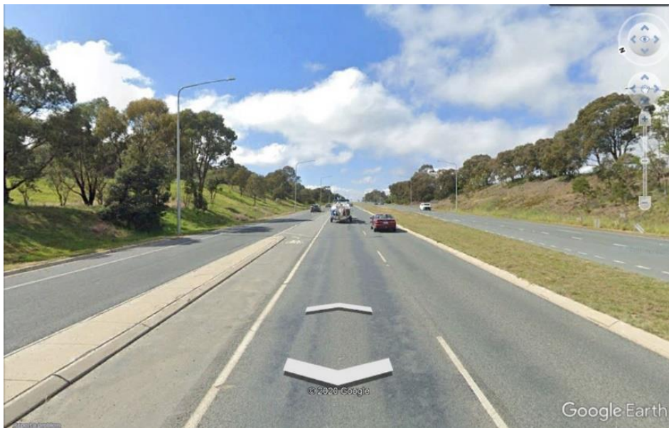
Figure 3: William Hovell Drive looking east from Coulter Drive (source: Google Earth)
