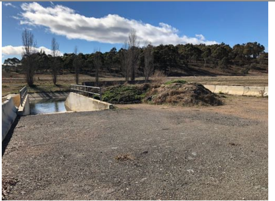
Ngunnawal GPT and stockpile
