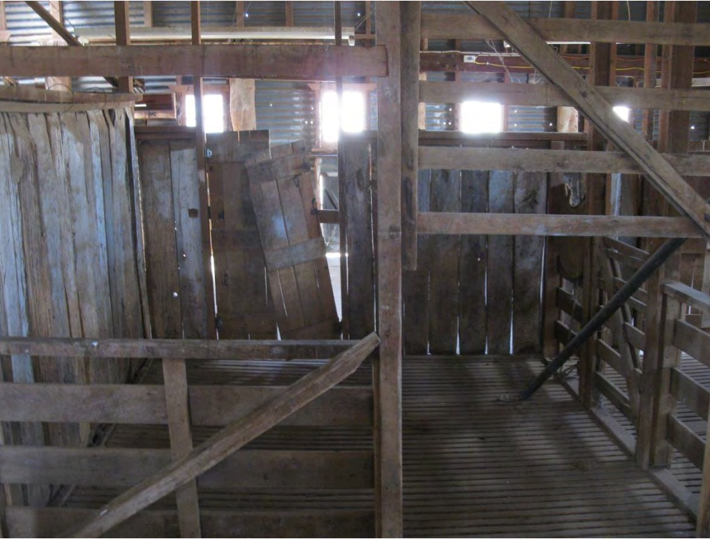
Plate 6. sheep pens showing lift gate and batten floor – note slab walls to left and rear
