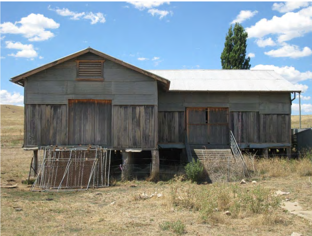
Plate 2. South elevation note sheep ramp on right
