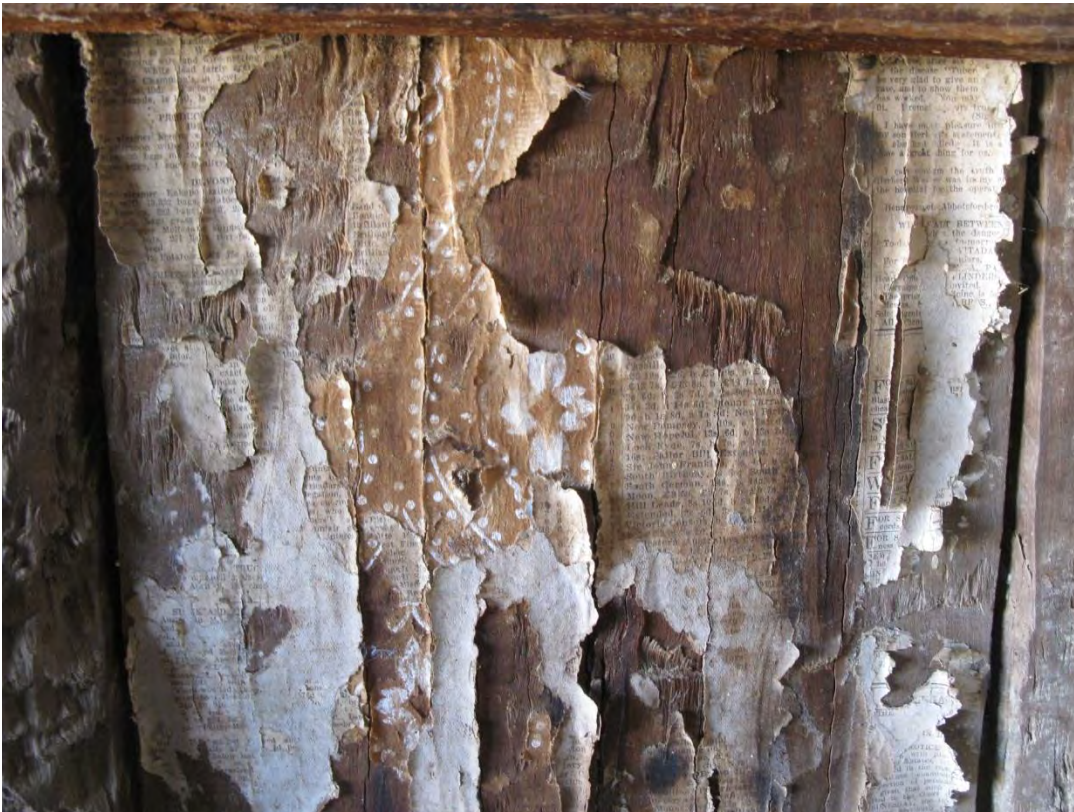
Plate 9. wallpaper overlaying newsprint on recycled timber slab walls
