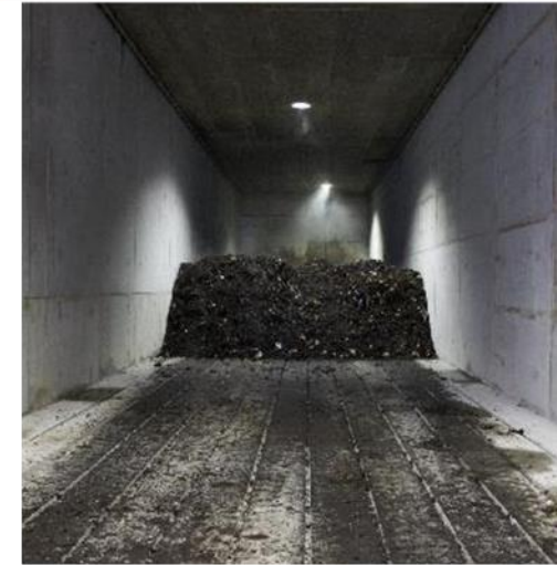
Example tunnel partially filled with compost
