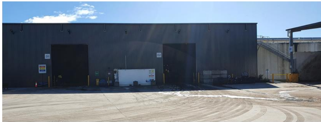
Example receival building
