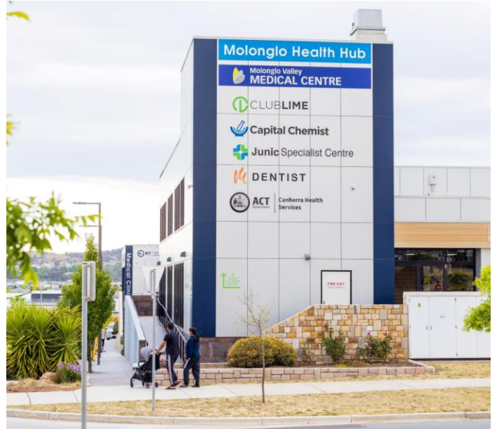
Figure 9: Molonglo Health Hub in Coombs, containing Canberra Health Services at Molonglo and Molonglo Valley Medical, and other ancillary health facilities
