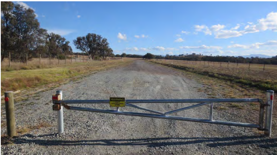
GRAVEL ROAD ADJACENT BLOCK 11
