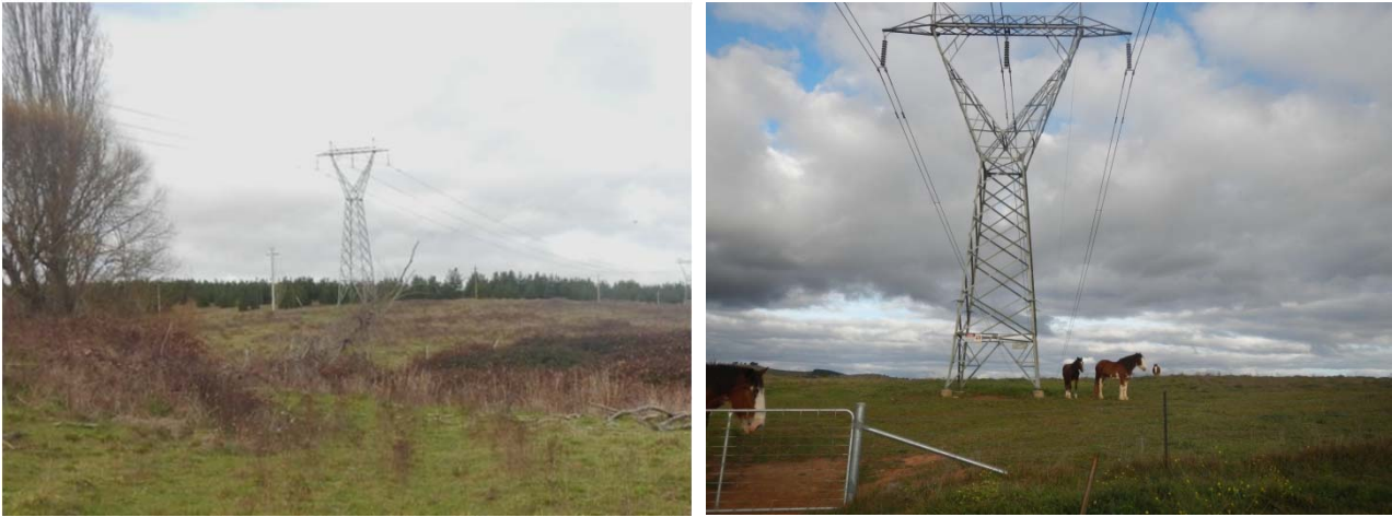
Figure 2.4 – Existing Steel Towers
