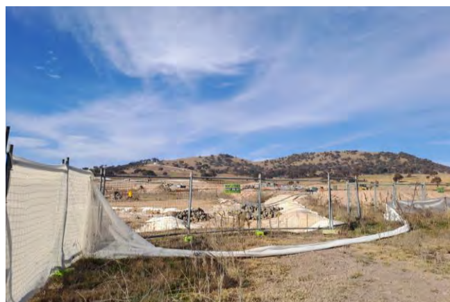
Photo 6.12 View of the South Jerrabomberra Village construction site, facing southeast
