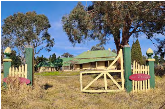
Photo 6.3 The dilapidated Hill Station cottage, Sheppard Street
