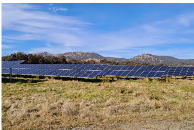
Photo 6.11 View of the Mugga Lane Solar Park and Environs Hills, facing southeast
