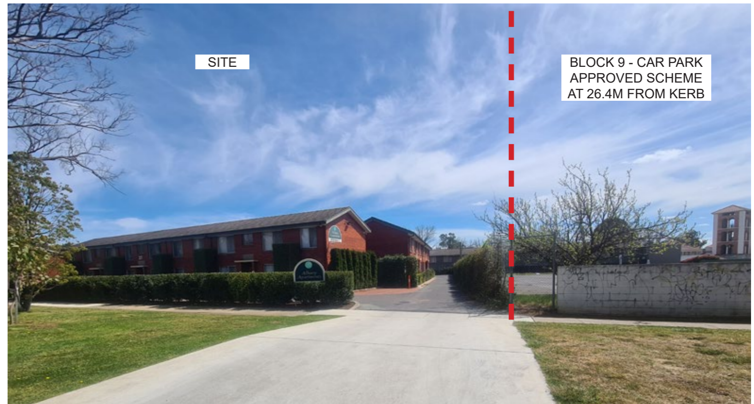
View of site interface with adjoining car park
