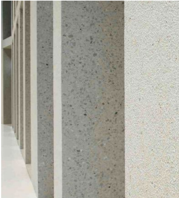
Warm, textural concrete elements
