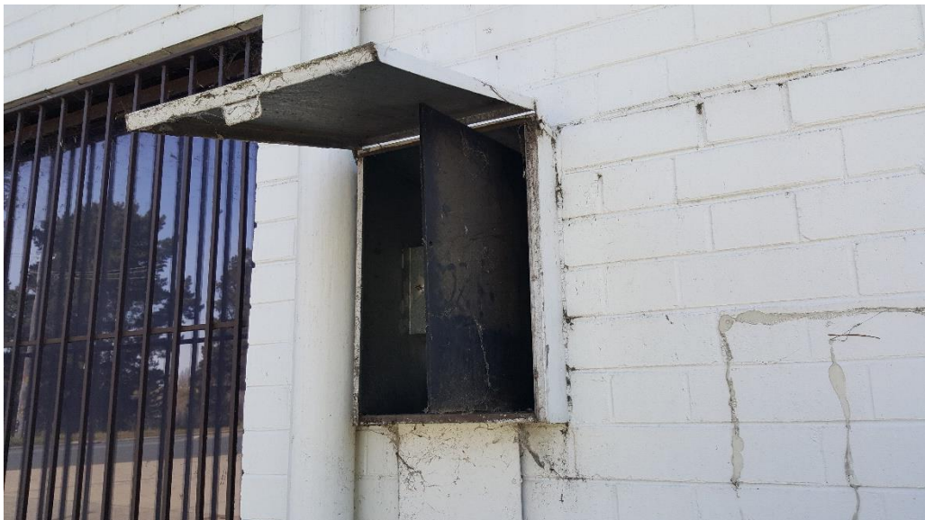
Photograph A10 Main Office Switchboard backing panel
