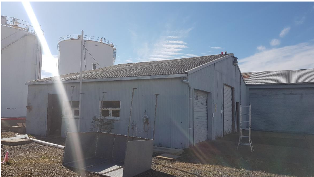
Photograph A6 Store shed (front) Corrugated sheet roof
