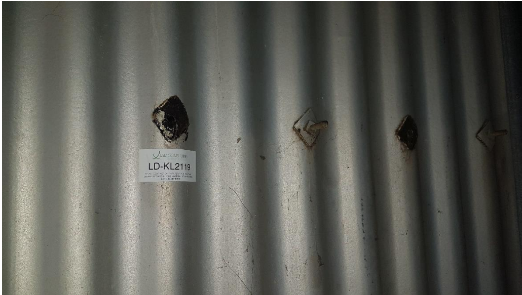
Photograph A5 Store shed (rear) Bitumen layer beneath tin screws
