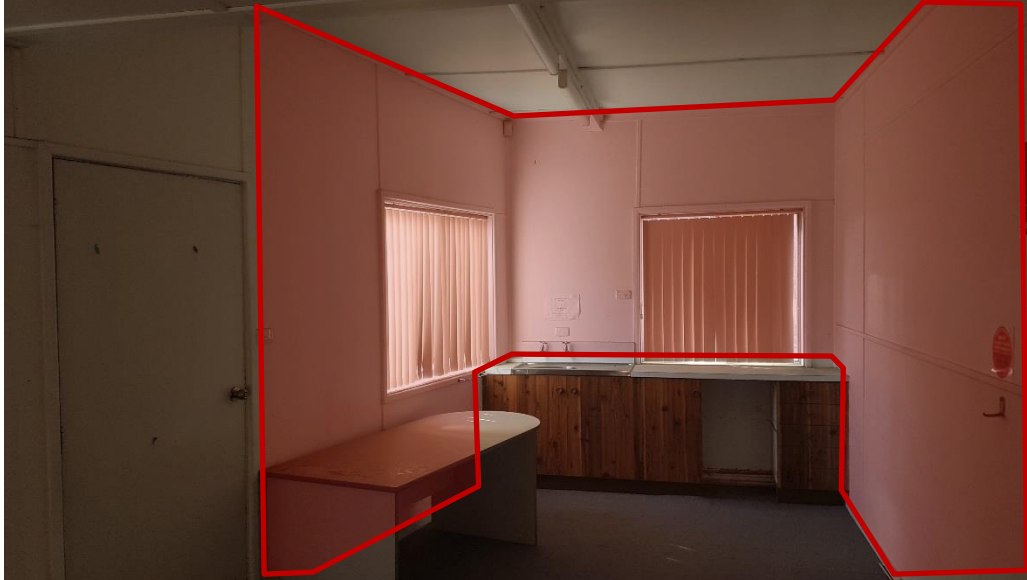
Photograph A1 Store Office Wall sheet to SE end of building
