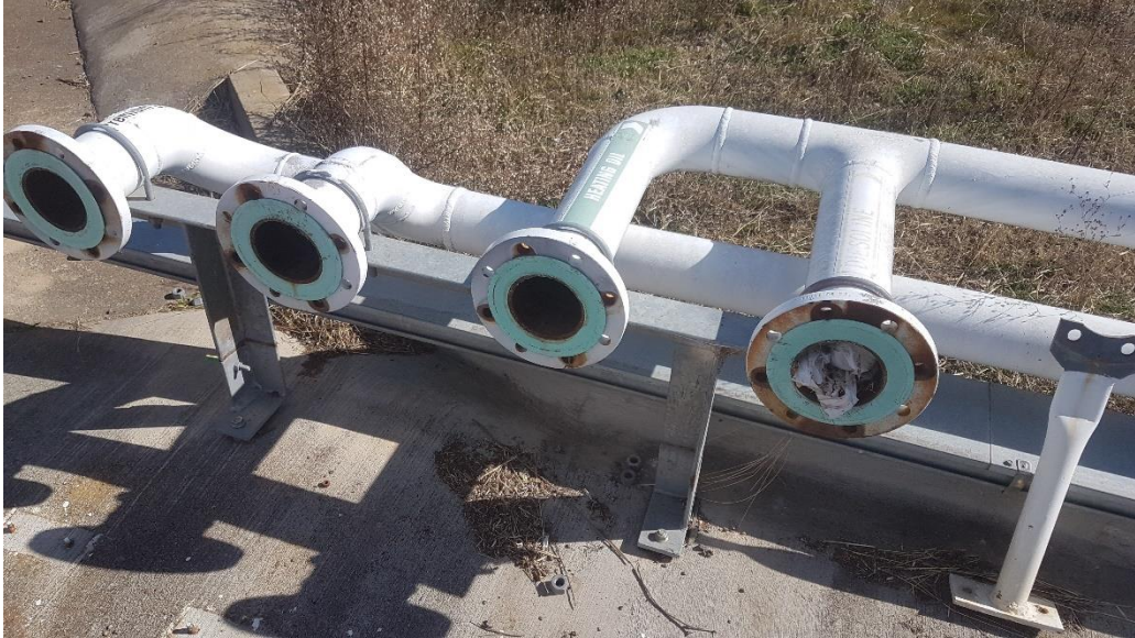
Photograph NA3 Pipe flange joints adjacent road bridge
