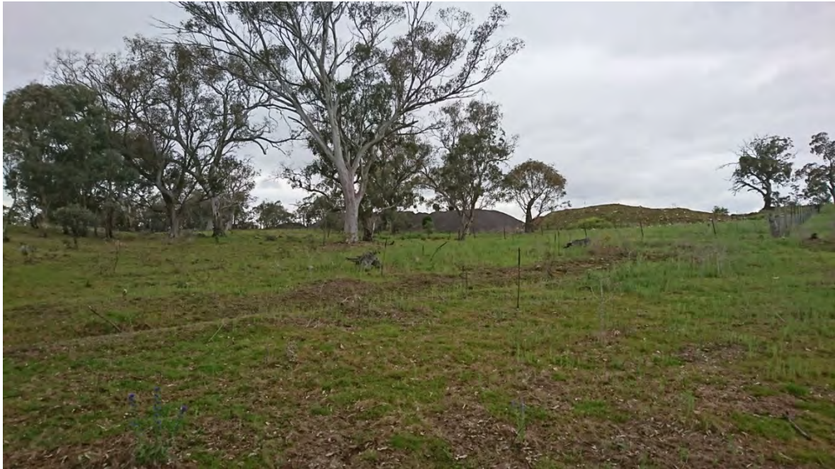
Photograph 1.1 An excavated drainage line in Area 1
