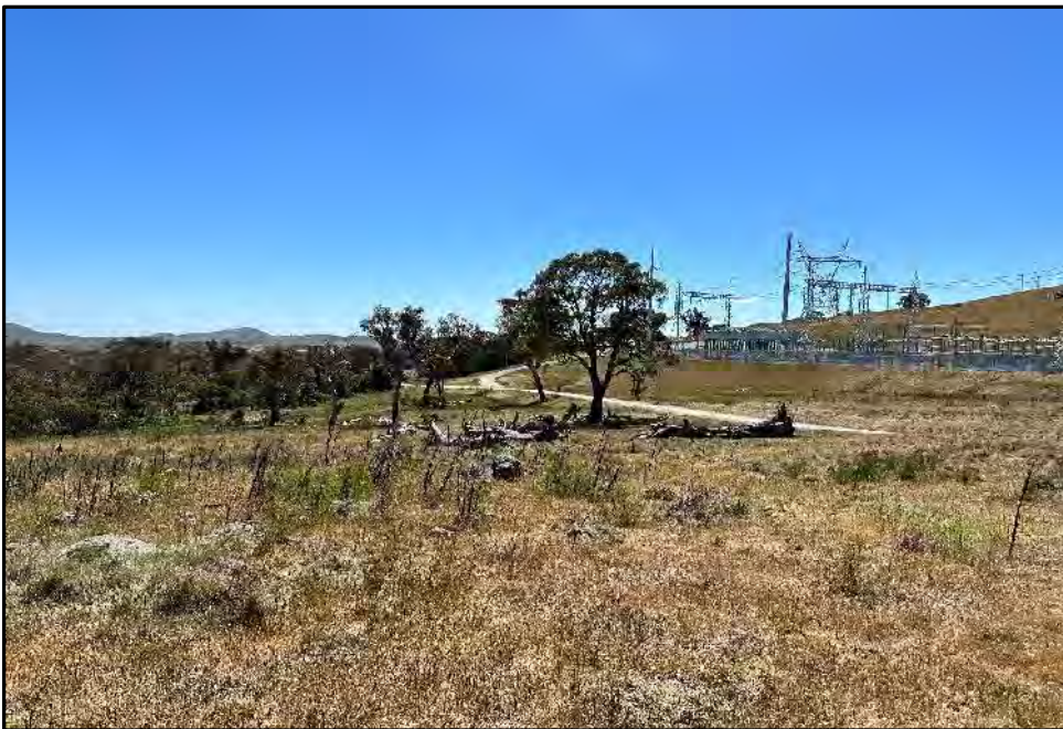
Photo 24: View of proposed tower 269A location, looking north-east
