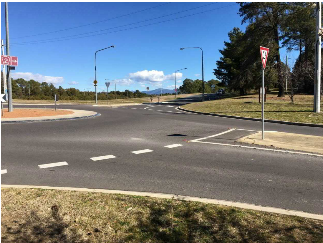
Figure 8 View of Novar Street roundabout looking west towards Dudley Street
