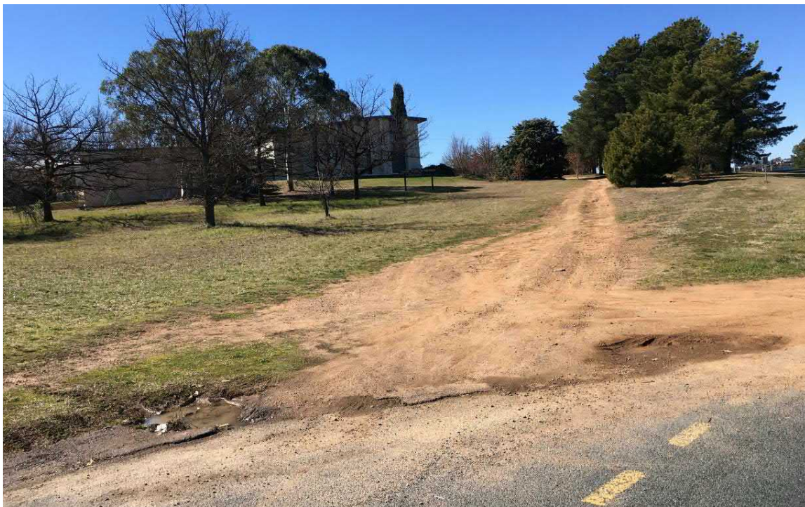
Figure 30 View showing the unauthorised access from Dudley Street to the Yarralumla Uniting Church car park
