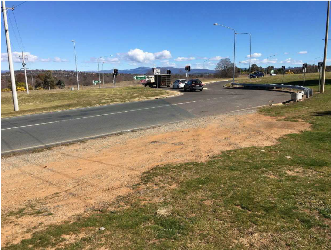
Figure 3 View of Dudley Street / Cotter Road intersection looking south from Dudley Street
