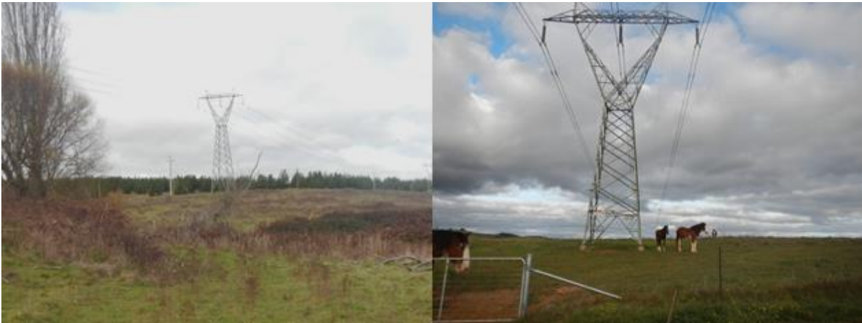
Figure 2.4 Existing Steel Towers
