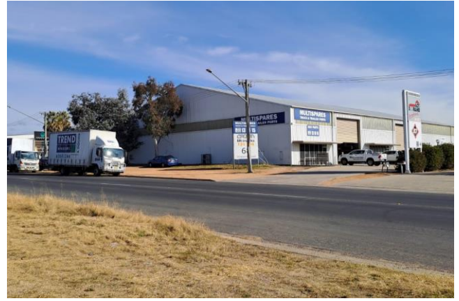
Photo 6.2 Typical built form within the Hume industrial estate
