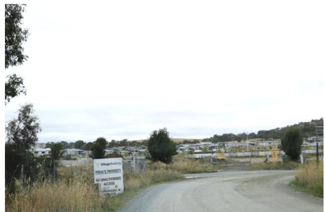
Photo 6.18 View towards the South Jerrabomberra Village construction site
