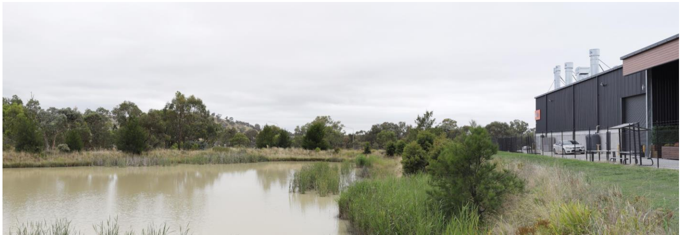
Photo 7.8 Viewpoint location 6: Couranga Crescent - existing view
