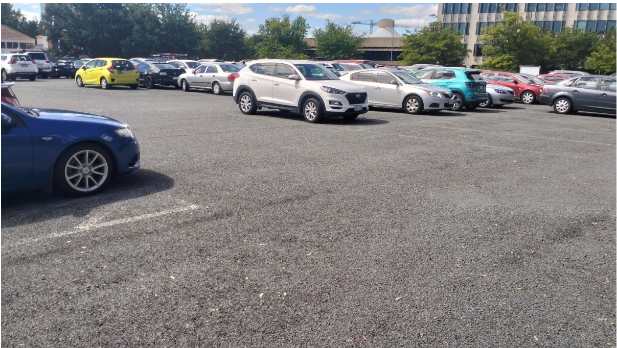
Photograph 2: Central area of car park facing east.
