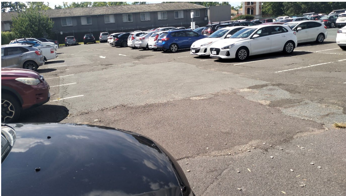
Photograph 4: Rear portion of car park facing north.
