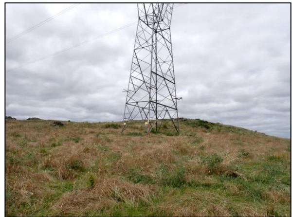
Plate 4. Tower 8, facing southeast of rocky sloping crest.
