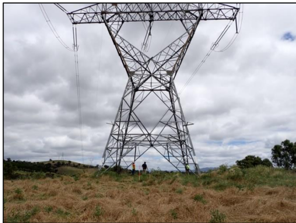
Plate 3. Tower 18, south facing over steep side slope above creek line.
