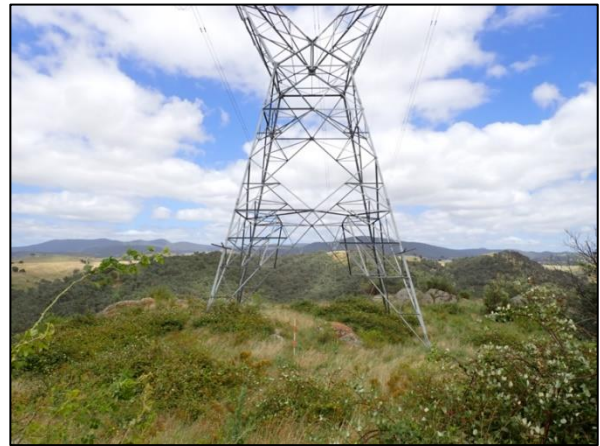
Plate 2. Tower 6, facing westward directly over banks of Murrumbidgee, on steep elevated hilltop, densely covered by blackberry bushes.
