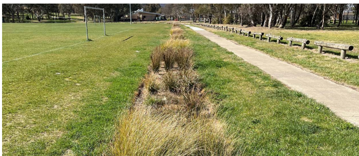
Bioretention swale at playing fields, Kambah, ACT
