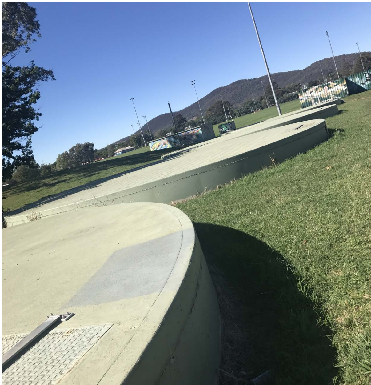
Stormwater harvesting tanks at sportsgrounds, Dickson, ACT
