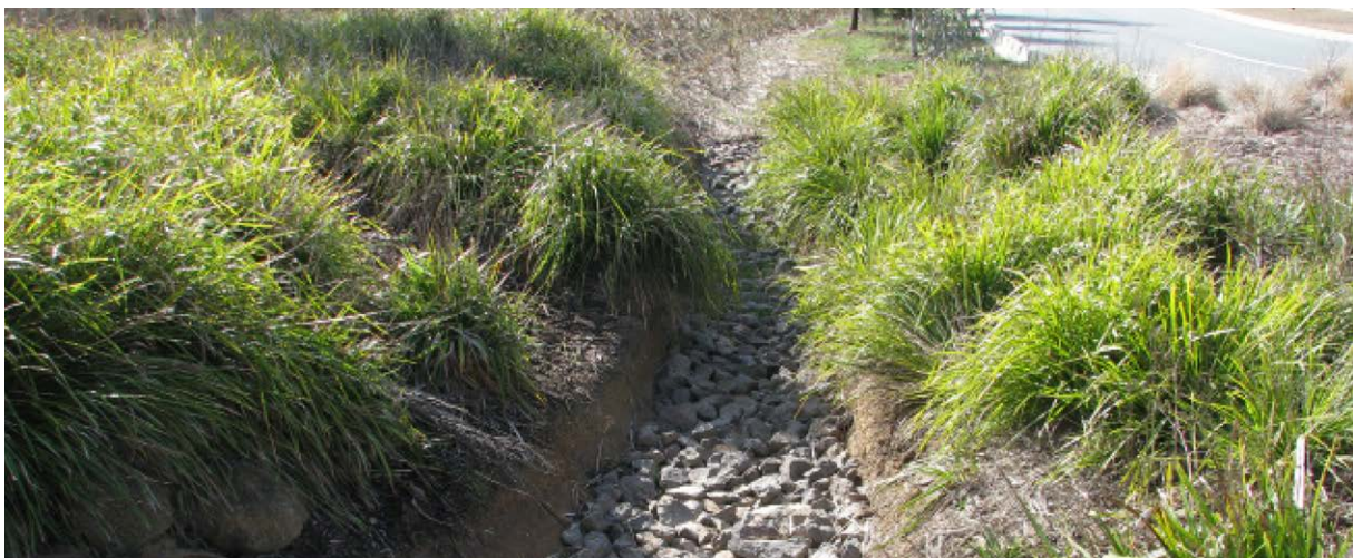
Rubble filter drain, Forde, ACT
