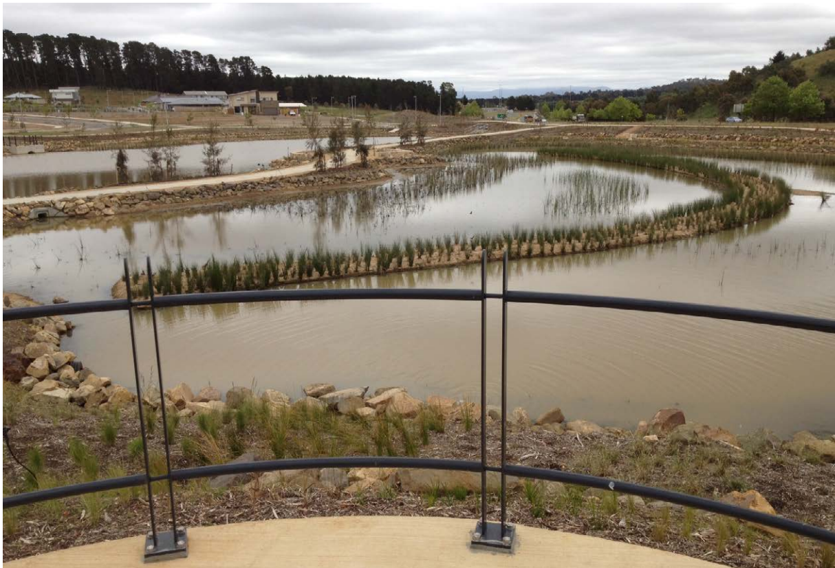
Newly constructed stormwater retention ponds near Abena Avenue, Crace, ACT
