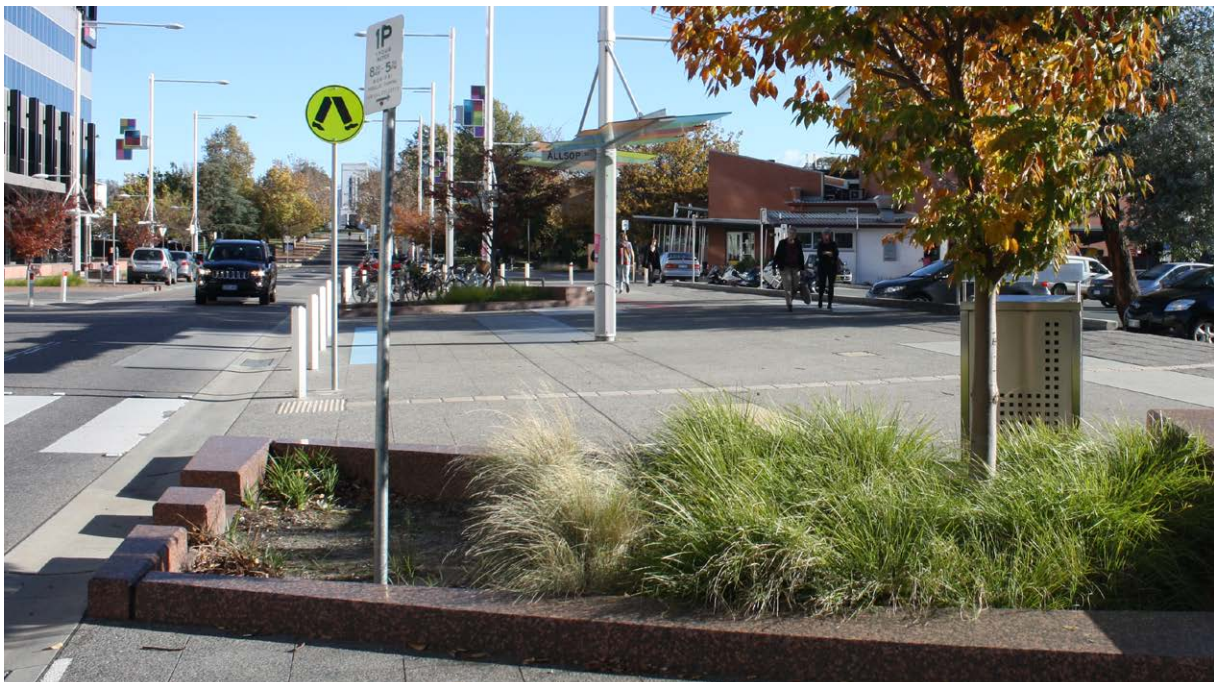
Castellated kerb and tree pit, Childers Street, Canberra, ACT
