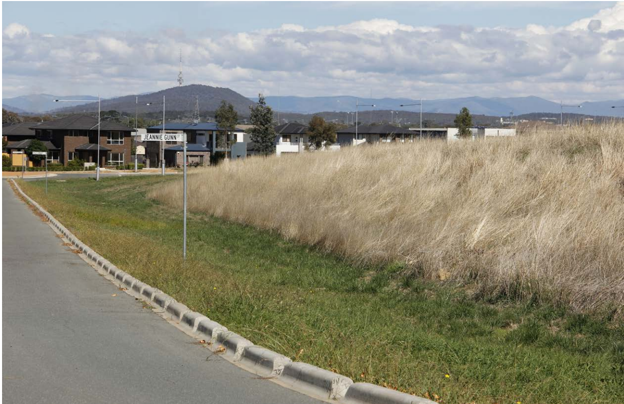
Castellated kerbs and grassy swale along Alec Hope Crescent, Franklin, ACT
