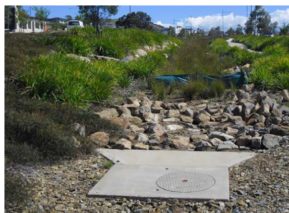
Water sensitive urban design reduces stormwater flow volume and speed
