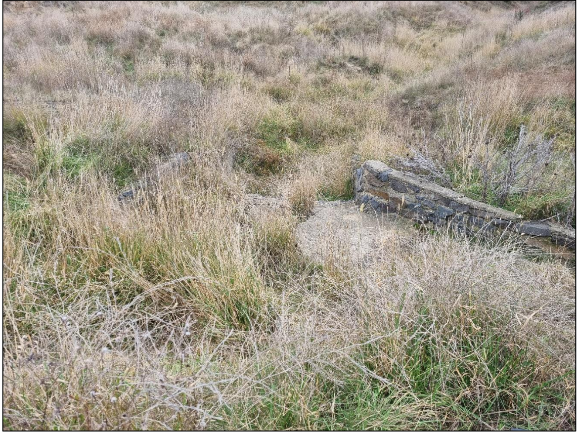
Figure 7-19 H/H4 - Erosion Control Measures
