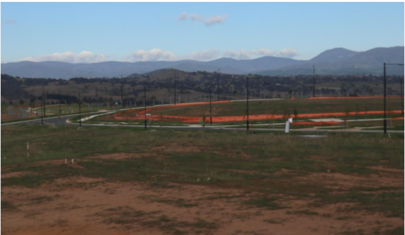
Figure 35. Whitlam Development. Erosion and sediment controls evident, as well as grasses, of variable coverage success, to restrict the transportation of sediment and velocity of water movement.
