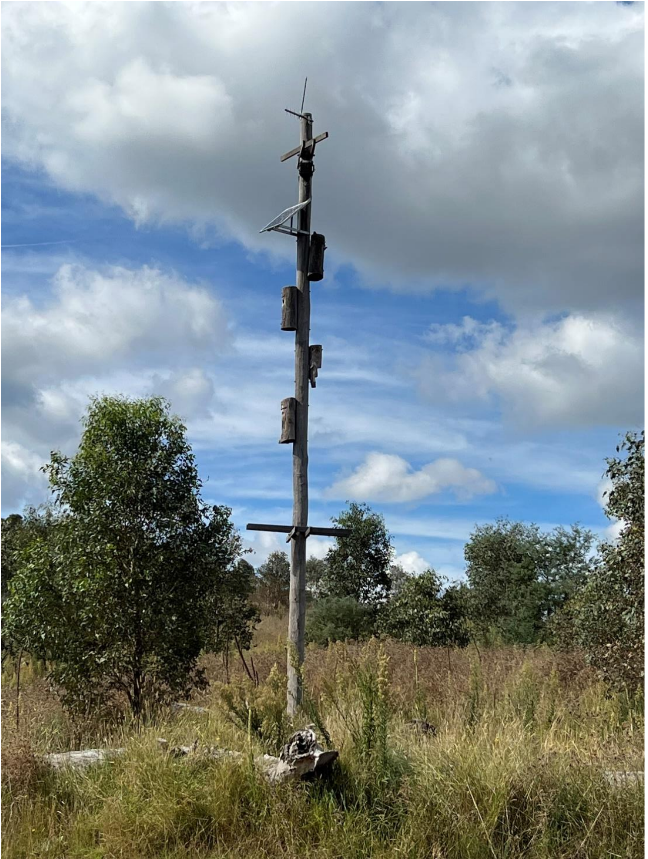
Figure 6. Barrer Hill Restoration site. Utility pole used for life support and wildlife habitat with hollows, bark and 'branches'. The maturing trees providing a diversity of habitat.
