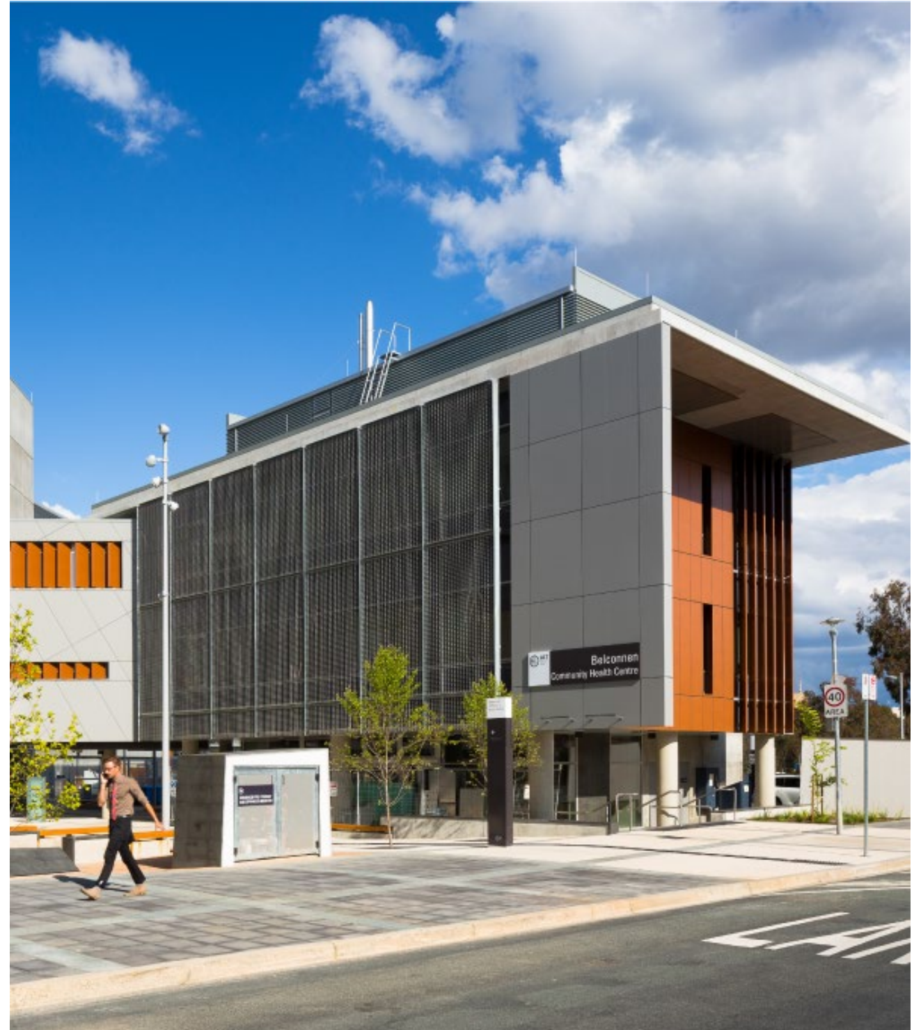
Belconnen Community Health Centre (image from Hindmarsh, hindmarsh.com.au)
