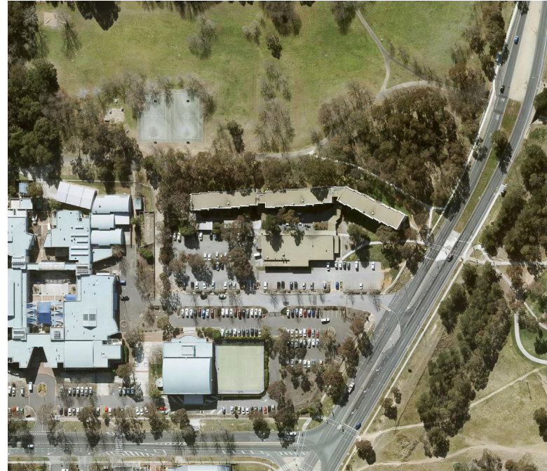
The site in 2014 (aerial imagery from Landchecker, 2025)
