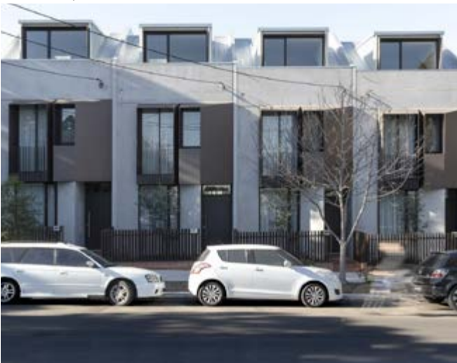
Photo 21: Using the roof form maximises internal amenity while minimising height and visual bulk. Portman Street Terraces, Zetland, Sydney NSW. Architect: CO-AP Architects. Photograph: Ross Honeysett
