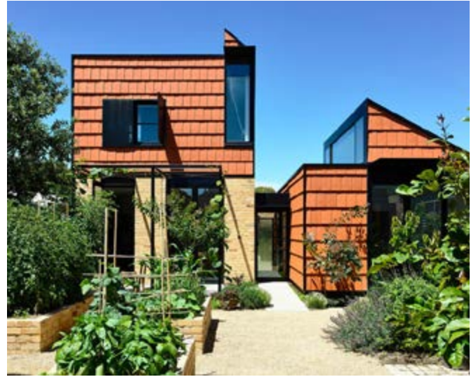
Photo 6: A high quality productive garden is integrated into the landscaping and is accessible from the buildings. Terracotta House, Melbourne Victoria. Architect: Austin Maynard Architects. Photograph: Derek Swalwell
