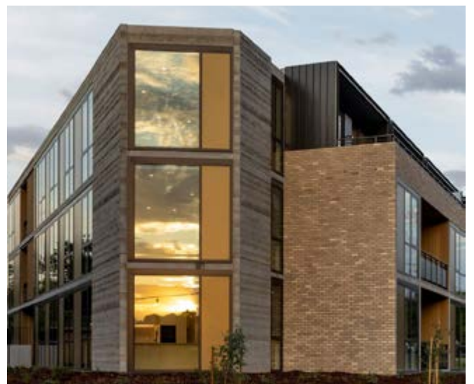
Photo 28: The positioning of the development on the street corner allows for a greater height and prominence. The Grounds, Ivanhoe East VIC. Architect: Architectus. Photograph: JWLand
