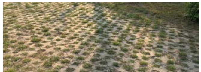
Photo 38: Permeable paving for driveways can effectively manage stormwater, reduce runoff, filter pollutants, mitigate urban heat island and enhance aesthetics.
