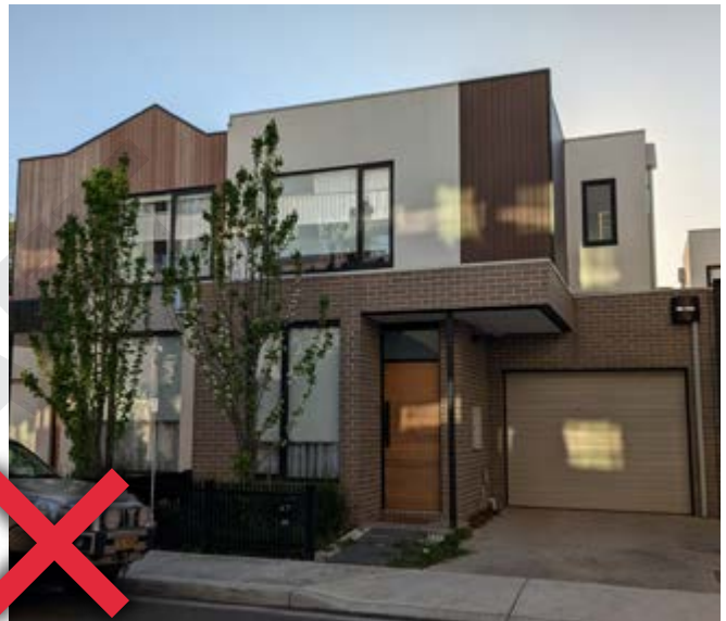
Photo 60: The excessive use of materials of a similar colour does not provide a quality visual outcome. Instead, the facade is too busy and dominates the streetscape.
