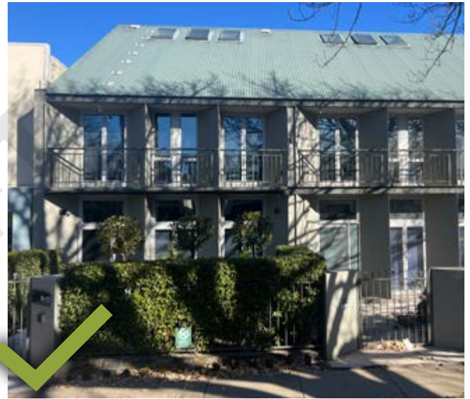
Photo 56: Simple saddle roof form. The skylights indicate a usable attic space in the roof. Turner Townhouses, ACT. Architect: Tzannes Architect
