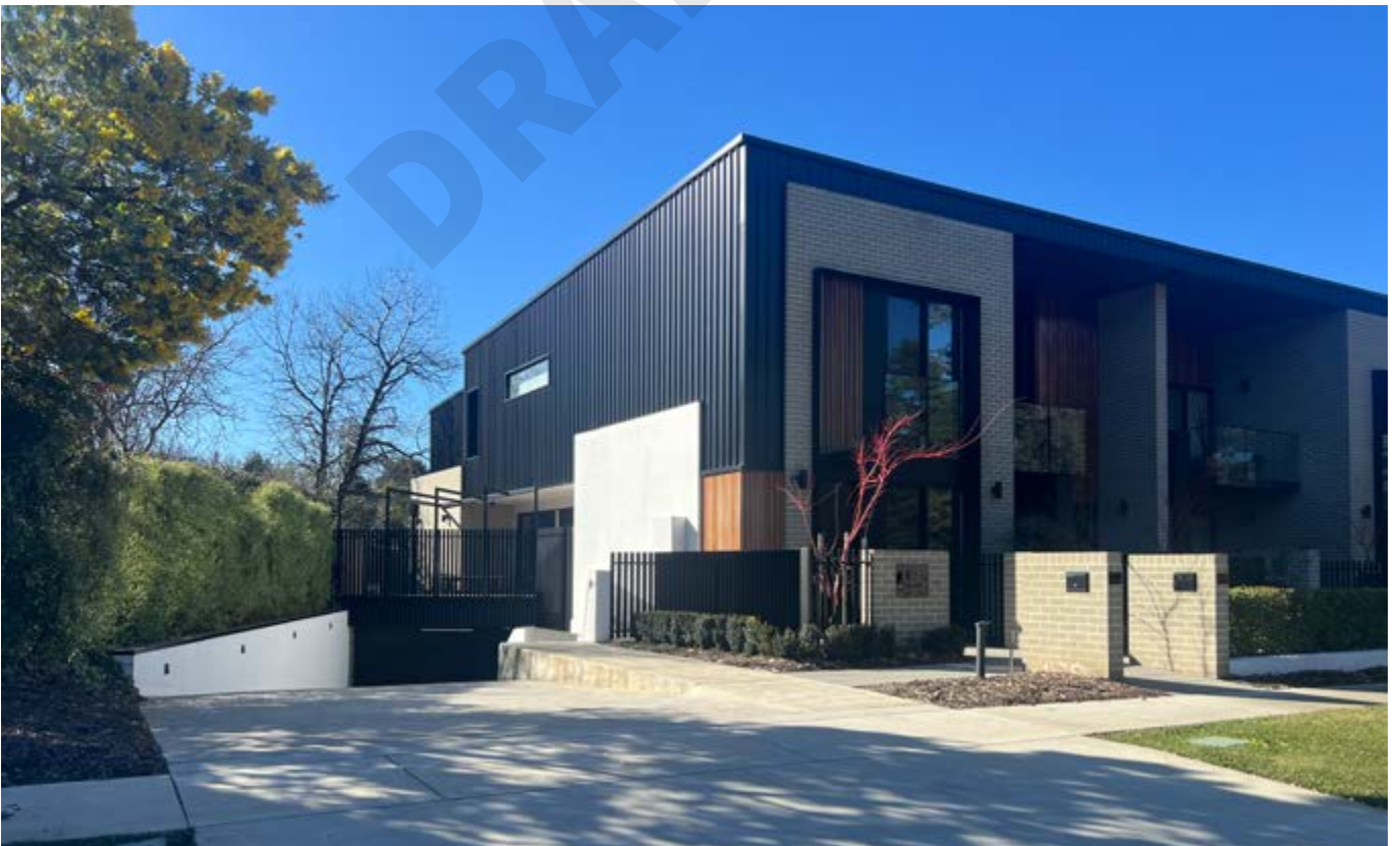
Photo 43: A sleeved driveway leading to a shared underground car parking area for the townhouse tenants. Haig Park Townhouses, ACT. Architect: DNA Architects.
