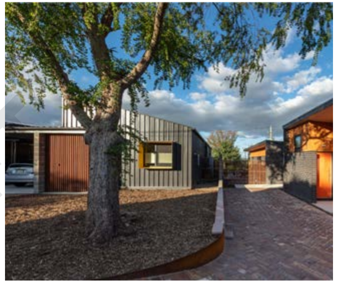
Photo 33: A retained tree can help to provide a focal point for the access-way, as well as reducing the urban heat island effect. The Village, Three Homes, Three Generations, Rivett ACT. Architect: Light House ArchiScience. Photograph: Ben Wrigley
