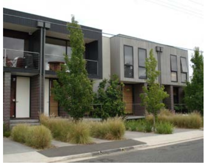
Photo 18: Architectural articulation and varied materiality can help to avoid a repetitive frontage. Townhouses, Geelong, VIC.
