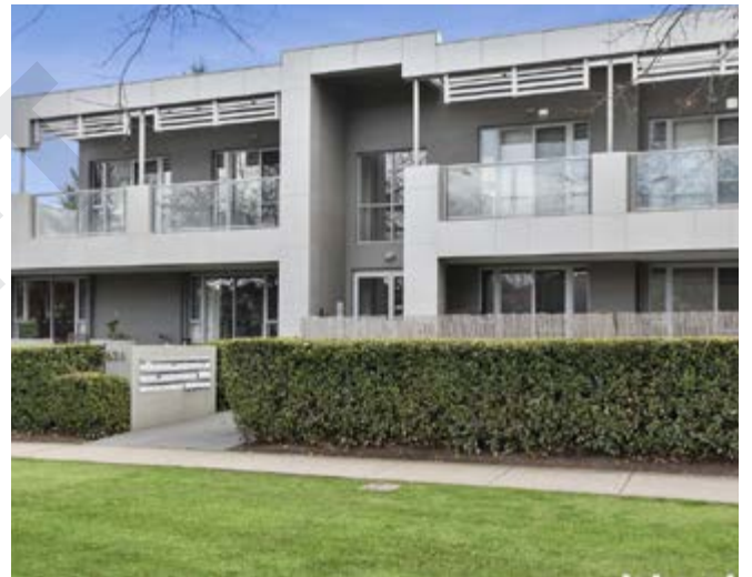
Photo 26: Landscaping and built form architectural articulation provide a clearly identifiable building entrance. Torrens Street Apartments, Braddon, ACT. Architect: Ring and Associates.
