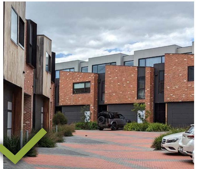
Photo 58: Articulation in roof form at the second floor. The upper level setback and modulation in form reduce the visual bulk of the third floor. Merri Green, Northcote VIC. Architect: Chamberlain Architects and Interiors
