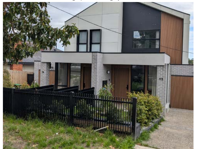
Photo 10: The ground level interface creates visibility to the streetscape and a relationship between both dwellings. Dual occupancy. Coburg North, VIC.
