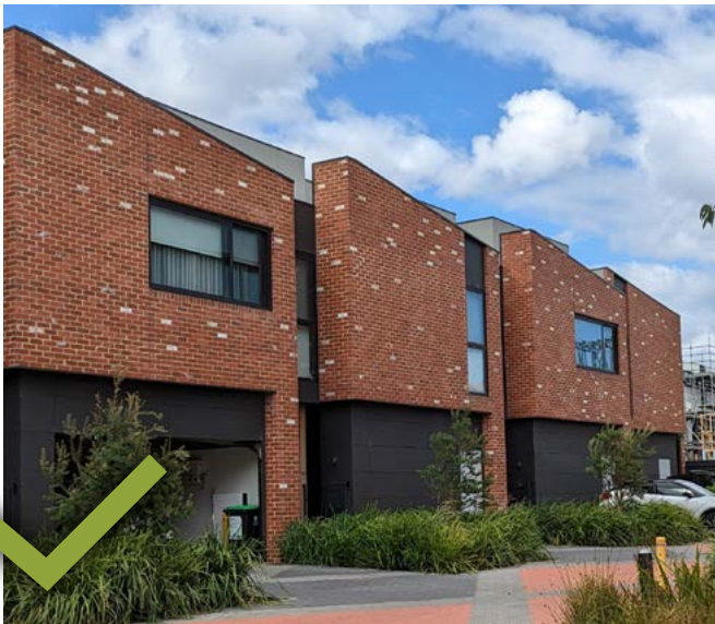
Photo 59: The use of simple materials such as brick and details such as black finishes and trimmings creates visual interest. Merri Green, Northcote VIC. Architect: Chamberlain Architects & Interiors.
