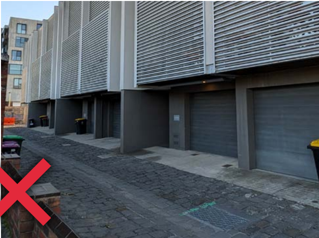
Photo 39: Garages without natural light and landscaping creates an unattractive and hostile urban environment which does not encourage other uses.
