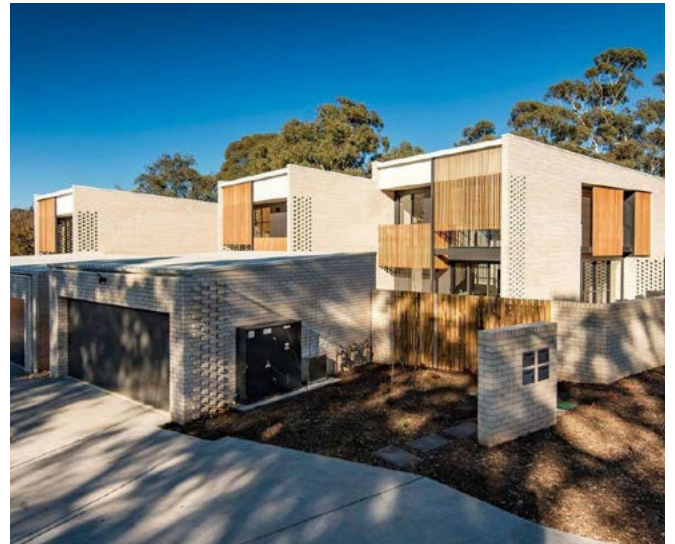
Photo 14: Louvres, screening and fencing maintain the privacy of the dwellings while also providing visibility. Holder Townhouses, Holder ACT. Architect: Stewart Architecture
